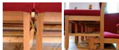
Left: Showing the H301 Keyhole Links, H702 Rubber Foot Ferrules and A118 Wooden Upholstered Kneeler, (Modified)
